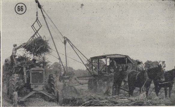
No. 65. Mule Powered Loader Which Replaced Hand Loading
