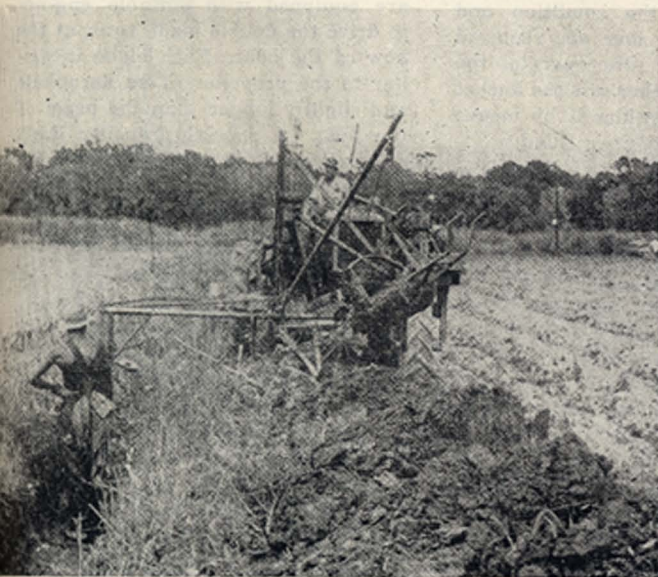
Photo No. 1 Thomson Cane Loader—Ditching Attachment.
