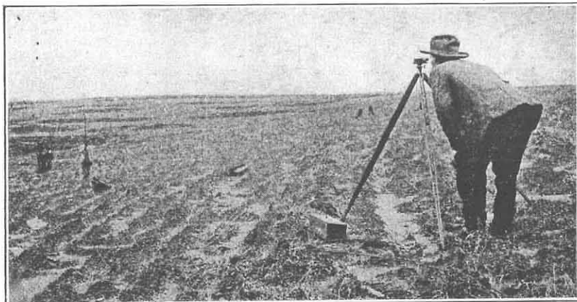
FIG. 5.—On a hillside the rows must run with the slope. They are laid out with a farm level and leveling pole, and the furrows are made with a plow
